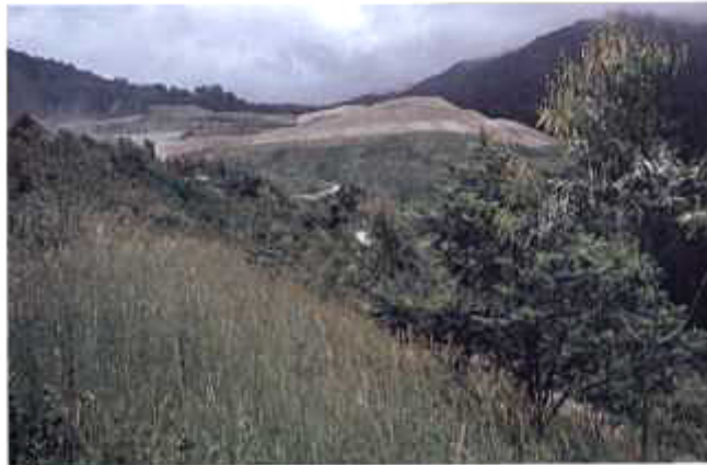
Plate 21.1: A good example of slope stabilization (foreground and middle background) at Mamat Copper Mine, with slopes in early stages of stabilisation in the background.
