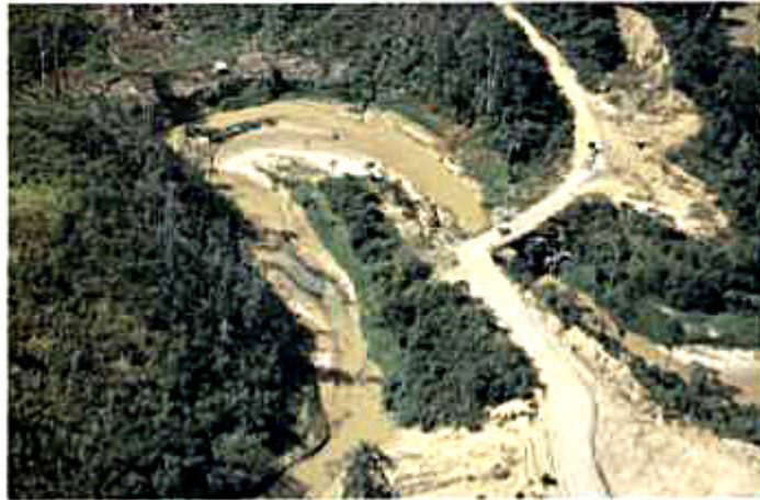
Plate 7.3: Areas disturbed as a result of road construction contribute to sediment load in nearby stream.
