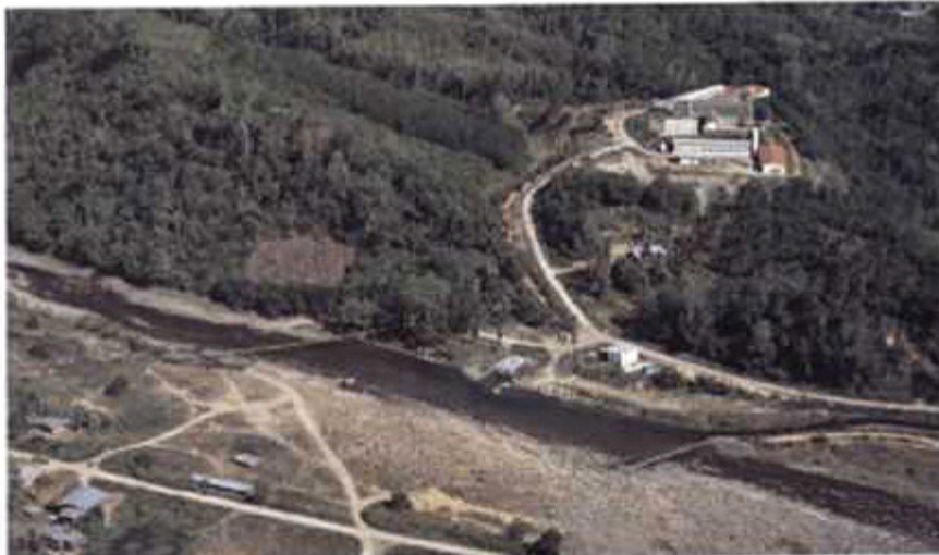
Plate 18.2: The intake (at centre) for water supply to Kudat has recently been constructed on Sg. Bandau, near Kota Marudu, upstream of the intake (at right) to the Kota Marudu Irrigation Scheme. Water for town supply is pumped up the hill to the treatment plant at upper right before being piped to Kudat. During low flow periods there is not enough water for both town water and irrigation. Irrigation is given priority and Kudat is short of water for extended periods.
