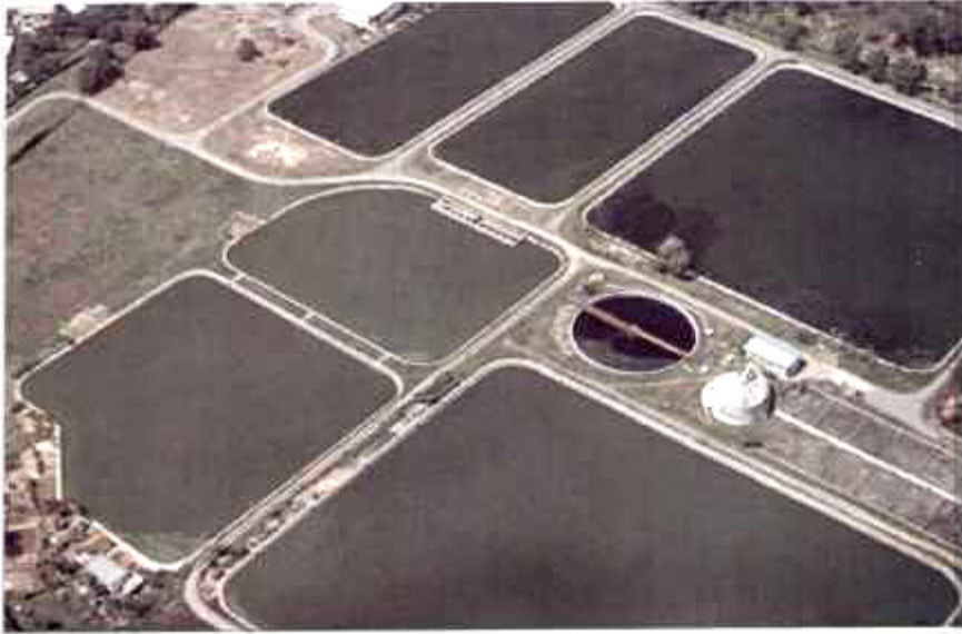
Plate 22.1: Urban sewage treatment using a trickling filter and lagoon system; Kota Kinabalu.
